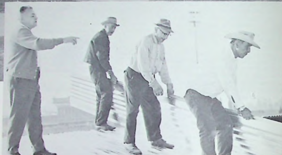
Portland Meadows roofing crew, right, puts aluminum sheet in place on barn roof. Meadows' Track Superintendent Jimmy Woodward, left, watches as Ed Denny, Joe Garbarino and "Blackie" Richard apply new roofing. Above, string of new roofs add improved look to Meadows backside.
